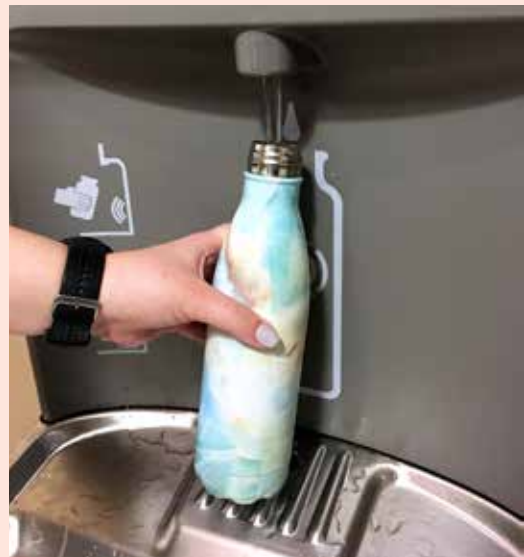
Newly installed water fountains with water bottle filling stations
